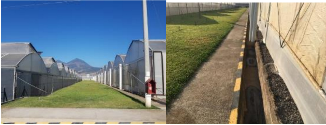
FIGURE 5 Greenhouse containment walls (Source: Dossier section 1.0, 2.0).
