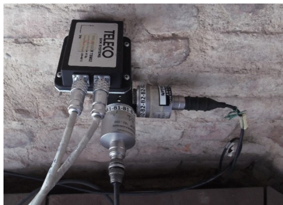
Figure 2.7: San Prospero bell tower: typical installation of piezoelectric and MEMS accelerometers.
