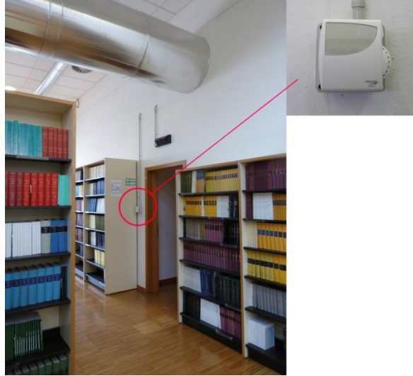
Figure 3. Pictures of a temperature sensor and its position.
