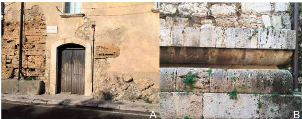
Figure 3. Remnants of Roman buildings in the urban centre of Isernia. (A) detail of the Roman wall circuit made of polygonal travertine blocks (to the left) resting on the Matese-Frosolone Unit dipping towards south (to the right); (B) detail of the podium in travertine of the Republican temple (major temple, III BCE) on which the cathedral has been erected.
