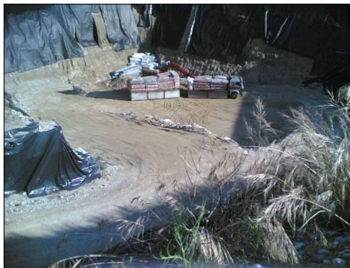
Figure 15-2: ACW unloading stage at an asbestos cement landfill site
