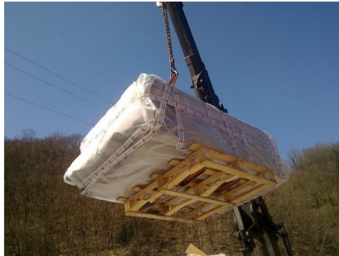
Figure 17-17: Removal of asbestos cement sheets
