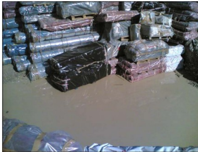
Figure 15-4: Asbestos cement packages transferred to special landfill
