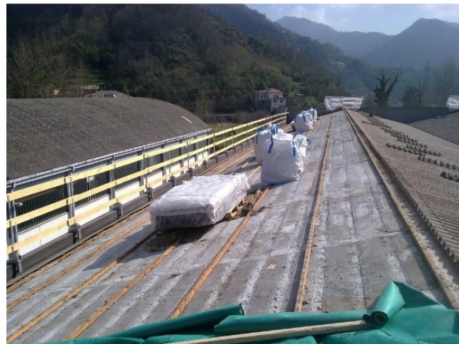
Figure 17-16: Removal of asbestos cement sheets
