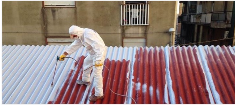
Figure 12-3: Method of decontamination: encapsulation
