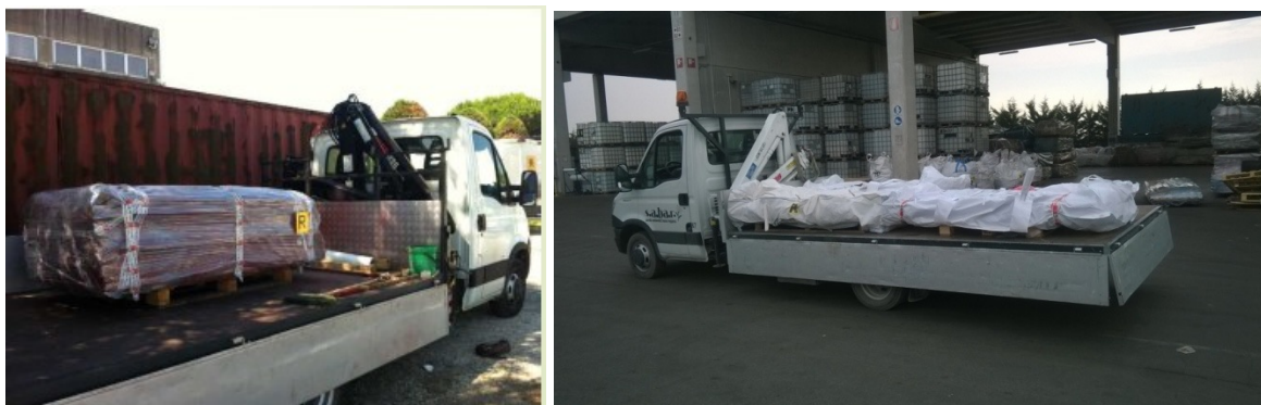
Figure 17-18: Transport of AC sheeting from the site to the storage facility
