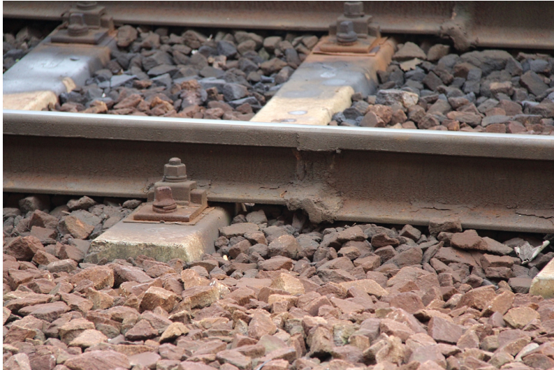
Figure 2.10: Thermite weld, in this case joining two different-profile rails: 50E5 (UNI-50) on the right, 60E1 (UNI-60) on the left.
