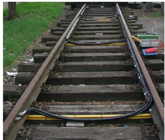
Figure 16.6: S-bond electric joint installation on test site.
