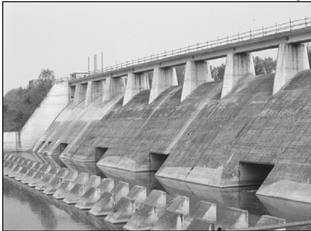
Fig. 8. Regulating dam of the “flow regulation system” of the River Panaro
