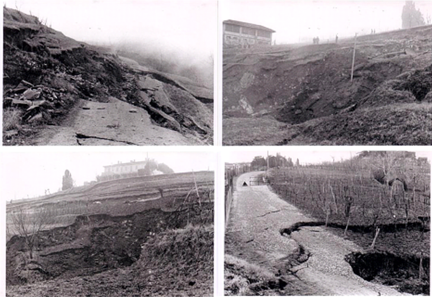
Figure 3: Pictures of the 1958 sinkhole.
