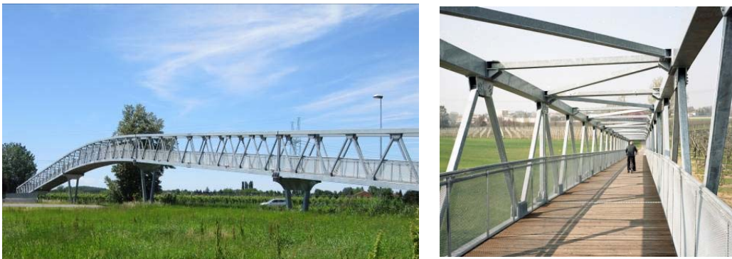
Figure 5. The Correggio Footbridge
