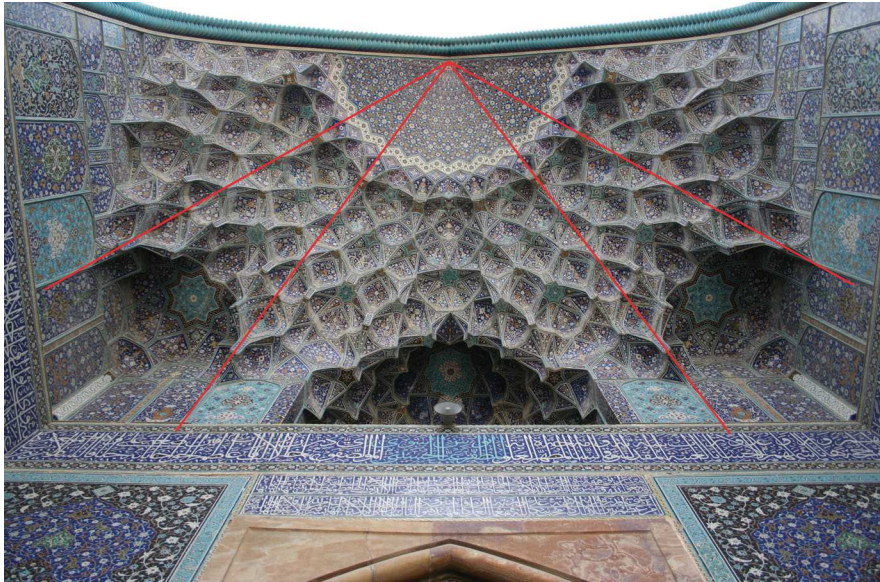
Fig. 12 Irregular star-shaped geometry of the muqarnas. Original photo: Patrick Ringgenberg, reproduced by permission
