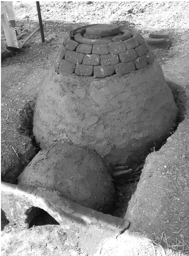
Fig. 5.25a. Constructing the single-chamber pit kiln.
