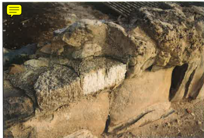
Fig. 2 – Top view of a partially dehydrated gypsum block in the Palace of Minos at Knossos (Crete). Note the white surface running parallel to the vertical face of the block (left). The maximum thickness of the white surface is about 4 cm.
