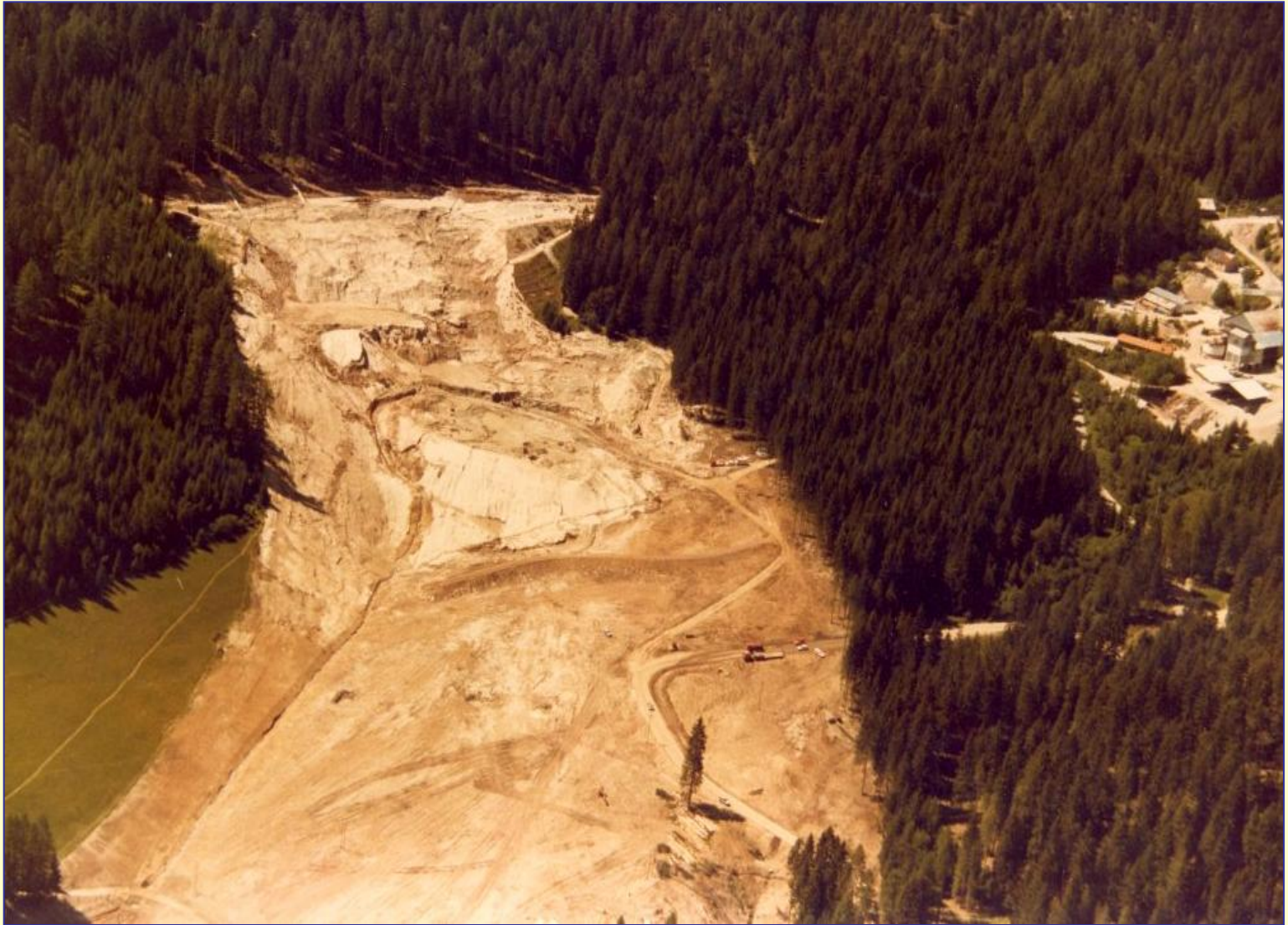
The upper Stava Valley soon after the tailings dams failure (July 1985)
