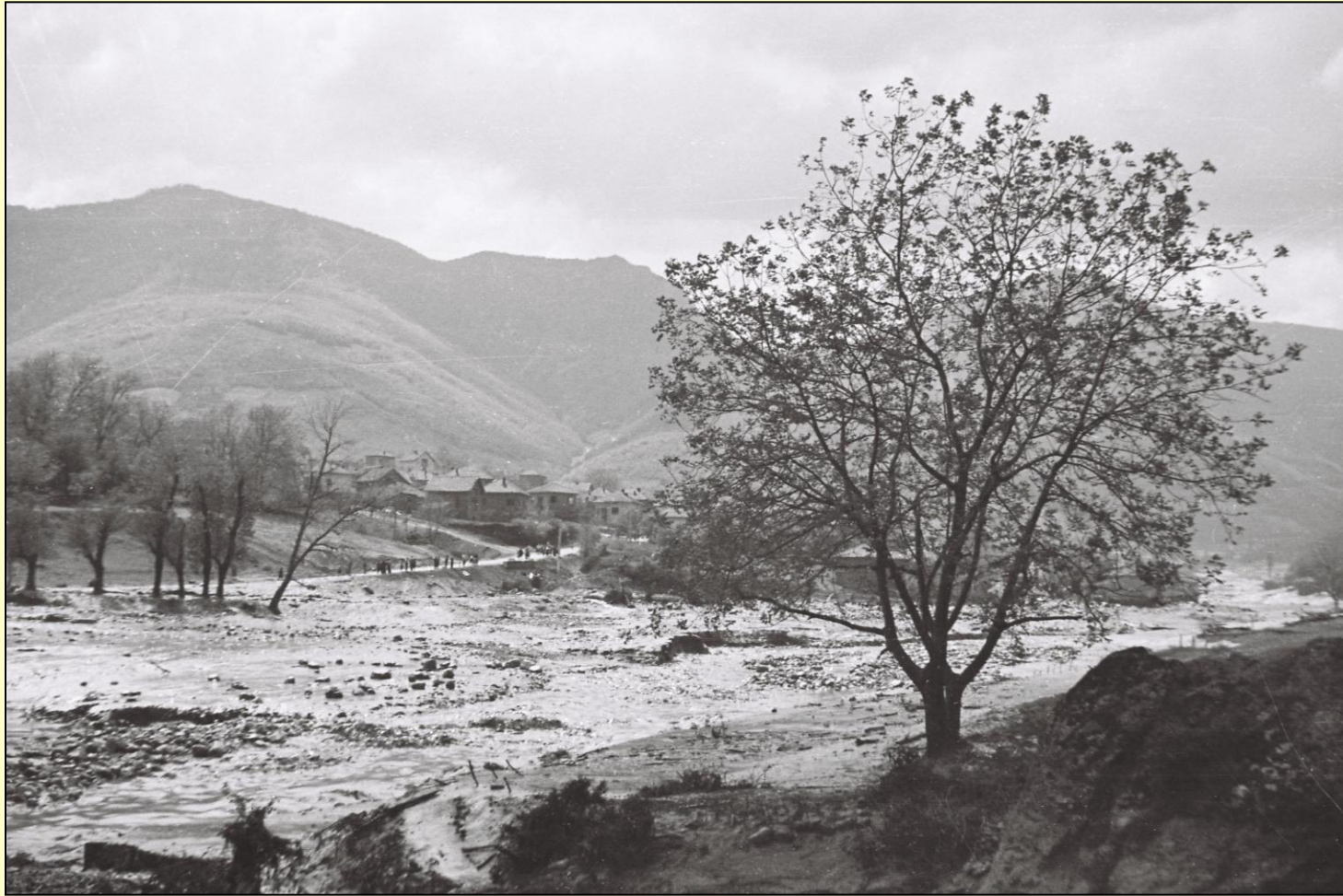
The Sgorigrad area soon after the collapse of the tailings dam (May 1966)
