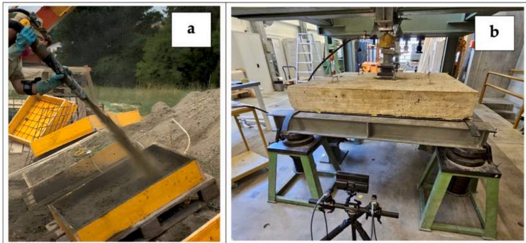
Fig. 2. (a) Shot-Earth projection process [9], (b) Test of a Shot-Earth slab.
