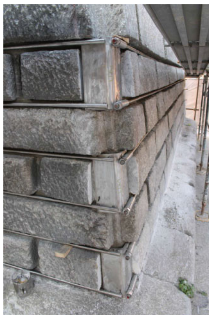
Figure 7. Post tensioned steel bars (B).
