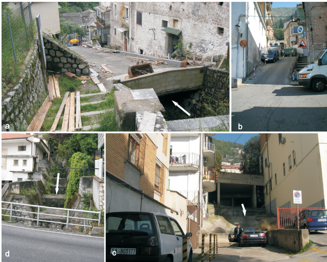
Fig. 9. Examples of hydraulic critical points in Sala Consilina: (a) and (b) the main stream is channelled underground; (c) the stream re-emerges but its bed has become a road; (d) the stream has a very small cross-section and is completely surrounded by houses.
