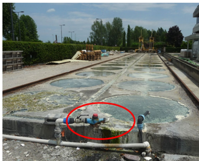
Fig. 1 Open-air pools for mud maturation in spa A (a) and in spa B (b). The yellow arrows and the red circle indicate the points from which thermal water flows and feeds the pools
