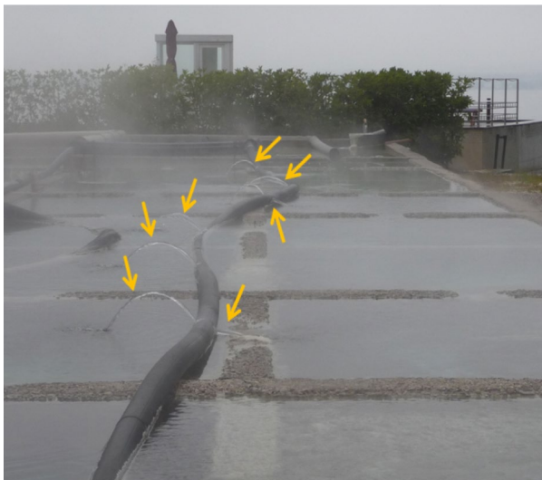
Fig. 1 Open-air pools for mud maturation in spa A (a) and in spa B (b). The yellow arrows and the red circle indicate the points from which thermal water flows and feeds the pools
