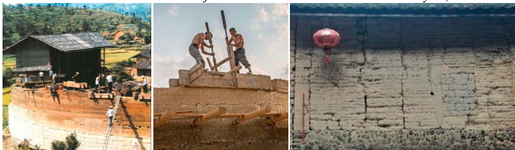
Fig. 2. Construction and pathology of Tulou (a) Source: Fujian Tulou (b) Source: Ramming Technology of Hakka Tulou
