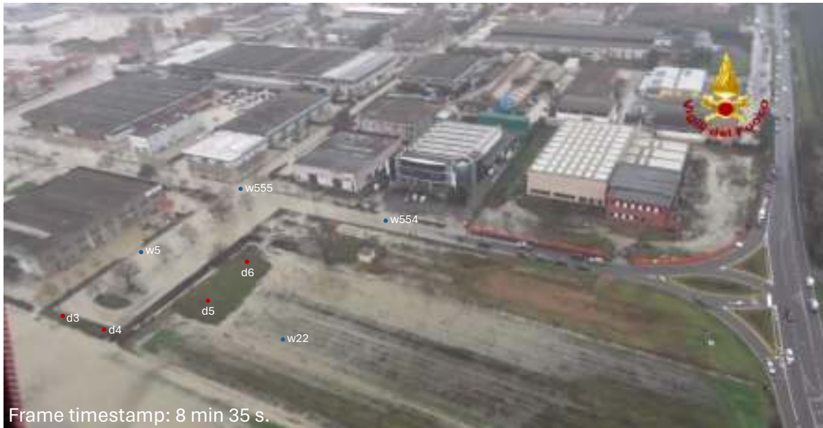
Figure S29. Frame of the aerial videography taken by the “Vigili del Fuoco” Fire Department of Modena. Wet points are highlighted in blue and dry points are highlighted in red. The time reported in the frame is counted from the beginning of the aerial videography occurred on 20 January 2014 at about 11:30 AM.
