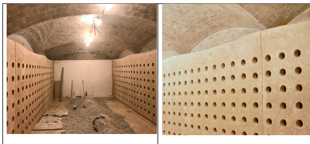
Figure 1. A wine cellar in Biel/Bienne, Switzerland: its walls are constructed using SE, capable of accommodating 400 bottles. These walls, along with the vault and pavement made of excavation earth rasillas, ensure perfect storage conditions for the wine ( www.pittet-artisans.ch , accessed on 12 January 2020 [8]).
