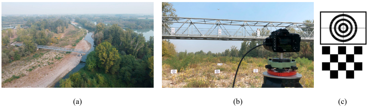
Fig. 1. (a) Wide view of the footbridge; (b) Detail on the monitoring setup; (c) target employed for the monitoring.
