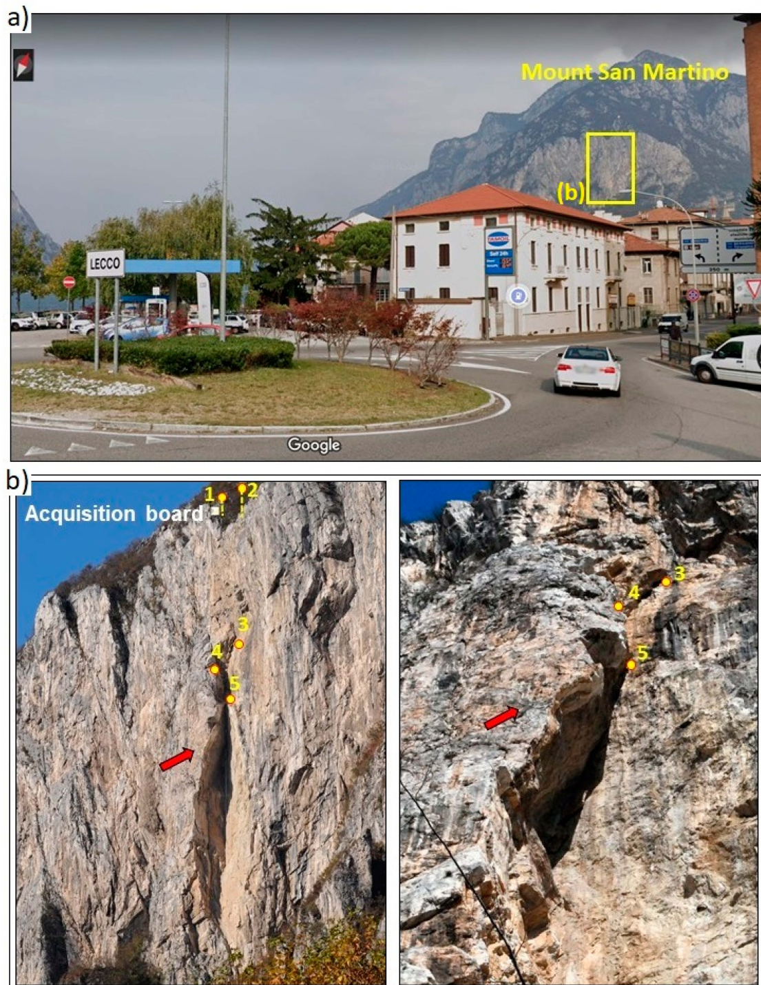
Figure 1. The study site in the southern part of Mount San Martino. (a) View of Mount San Martino from Lecco city. The yellow rectangle indicates the monitored area where the monitoring network was deployed. (b) Rock face with the positions of the five geophones and the acquisition board of the microseismic monitoring system. The red arrow indicates the partially detached pillar below Geophone 4.
