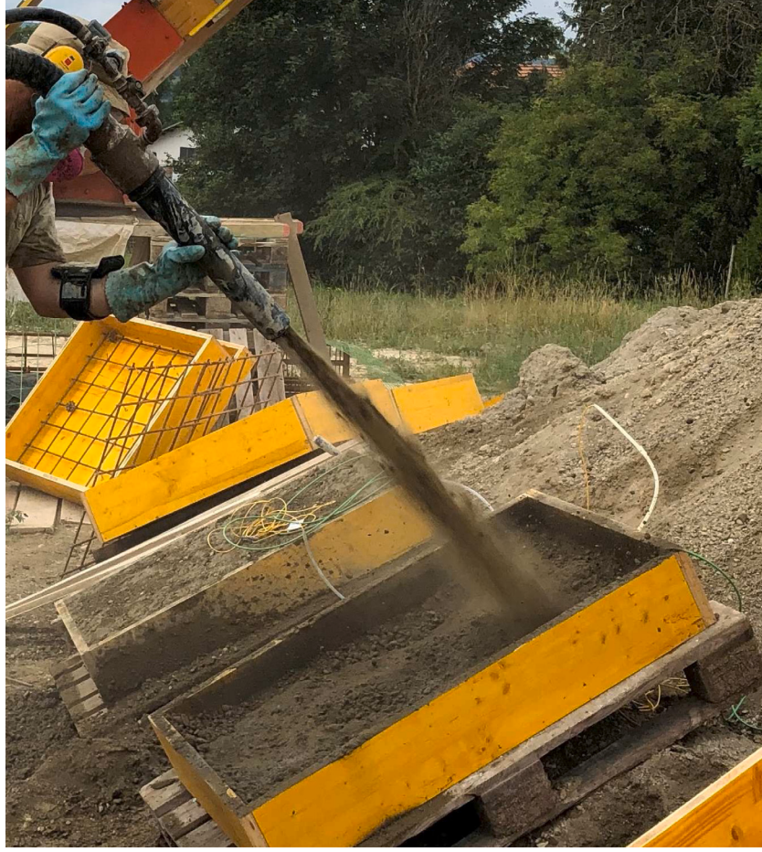
Fig. 1. In situ spraying process of shot-earth.
