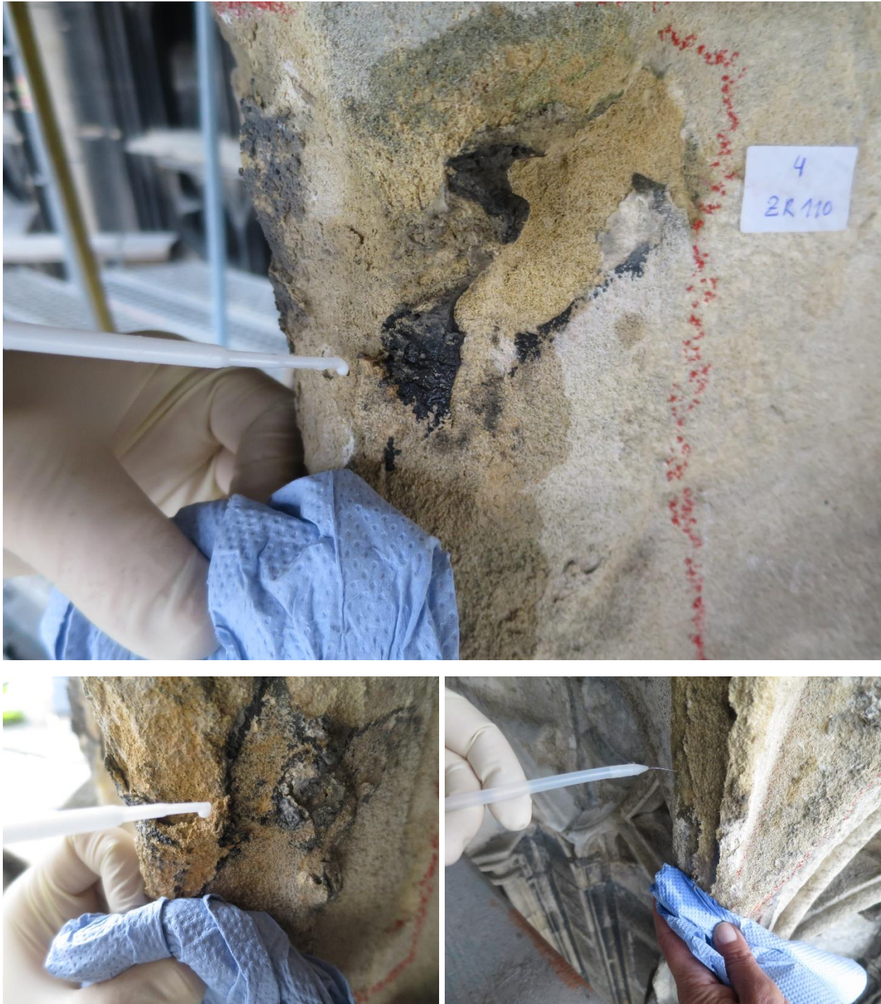
Figure S11. Intermediate restoration state, during the cleaning procedure and treatment application. The consolidants were applied by means of run-off methods with varying utensils.
