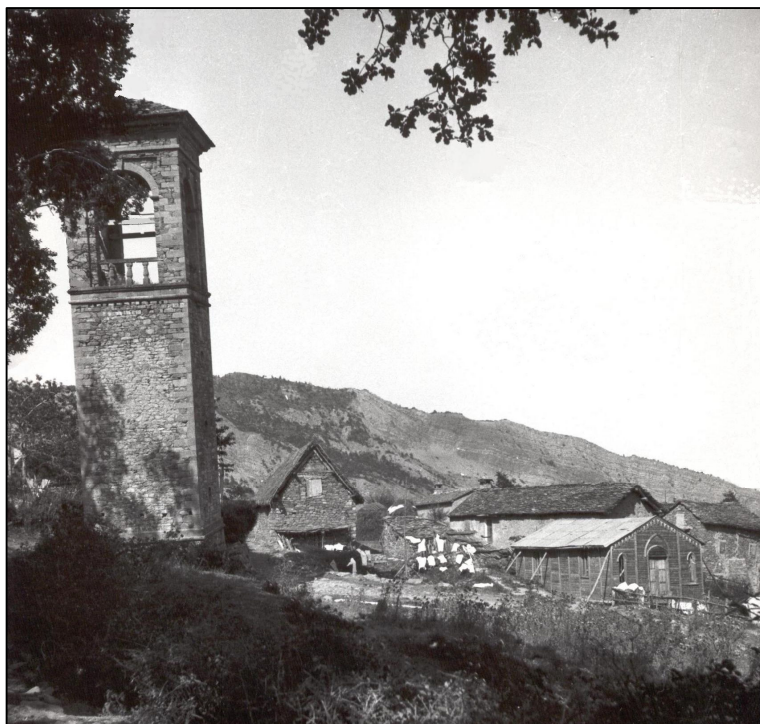
Fig. 8 Ground effects of the September 1920 earthquake in Febbio: the church tower has undergone considerable tilting owing to a seismically-induced landslide
