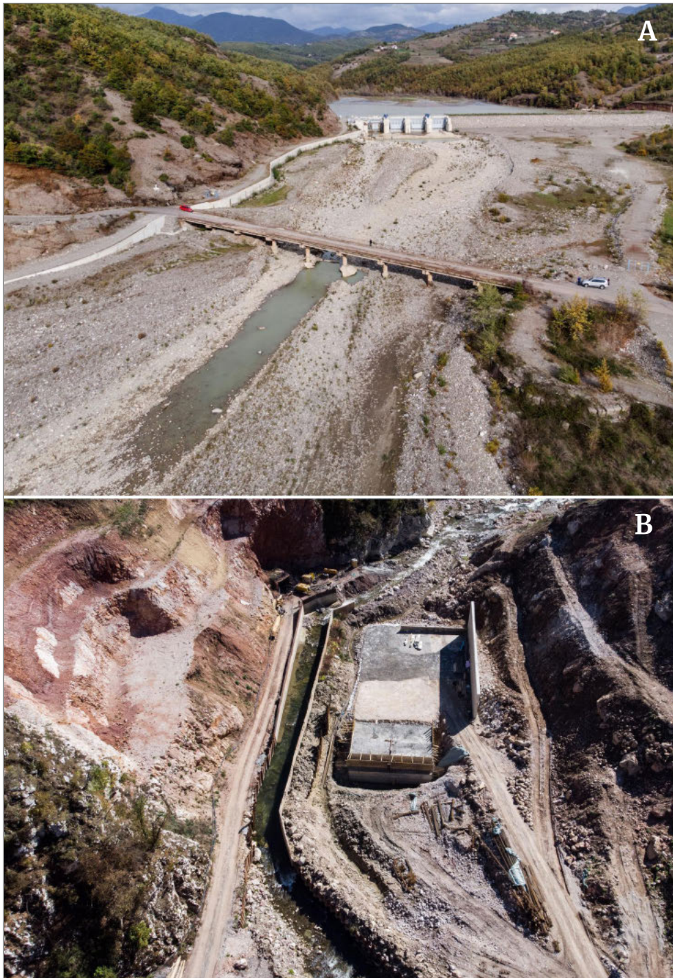
Figure 3. Nature after ‘green and sustainable’ renewable hydroelectric plants: (A) the dried, once great, Rapuni River; (B) a small dam on the Drinjaca River, showing huge destruction despite a so-called small scale hydro-power plant. Both photos by Amel Emric.
