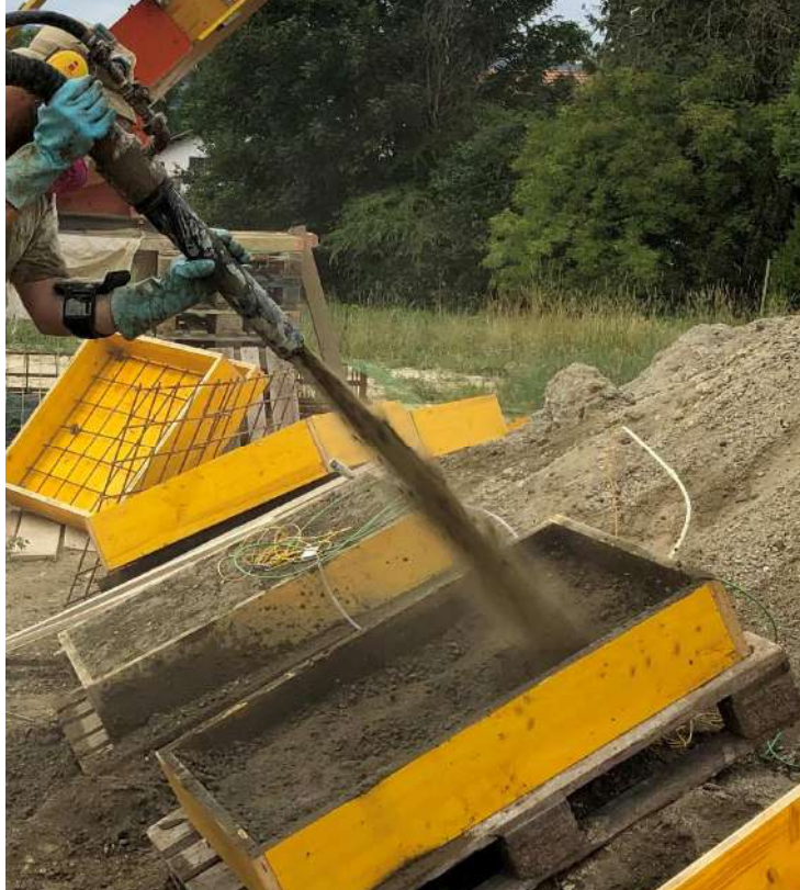
Figure 1: In situ spraying process of shot-earth.
