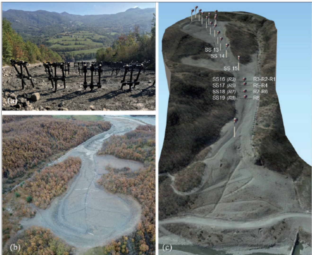
Fig. 6 – Field and aerial views of ground reshaping and MTS finalization as integral part of all other slope consolidation intervention. LEGEND: (a) Upslope to downslope field view. (b) Upslope to downslope aerial view. (c) Downslope to upslope aerial view with labels and relative position of monitored tripods (R1 to R8) and topographic monitoring prisms (SN13 to SN19)
