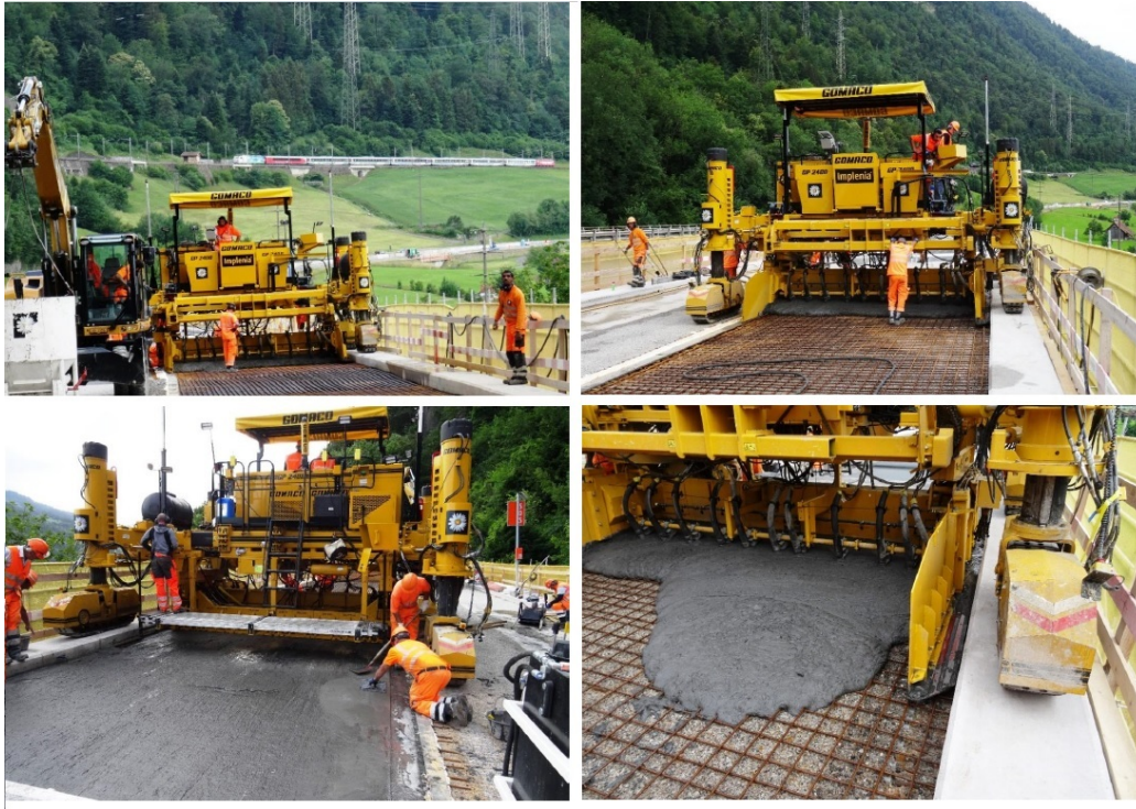
Figure 1: Switzerland 2018 [12] - Retrofitting of a bridge deck member by using a commercial UHPFRC
