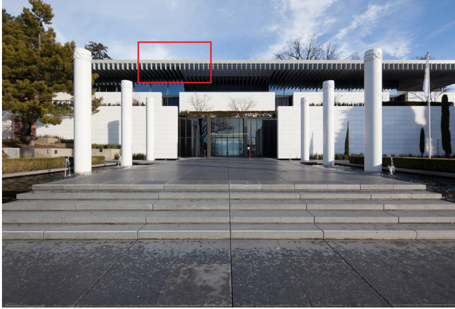
Figure 3.7: Photo of the Olympic Museum at Lausanne. The roof in UHPFRC was completed in 2013
