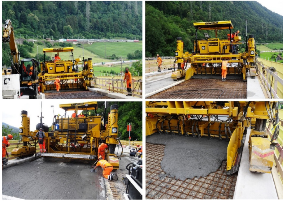
Figure 5.1: Switzerland 2018 [21] - Retrofitting of a bridge deck member by using a commercial UHPFRC
