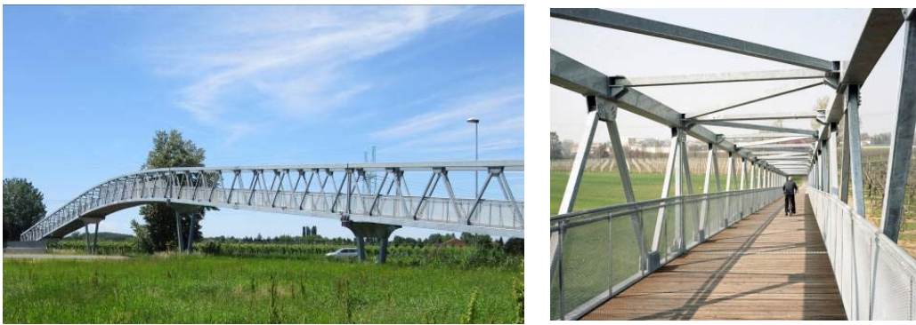
Figure 5. The Correggio Footbridge
