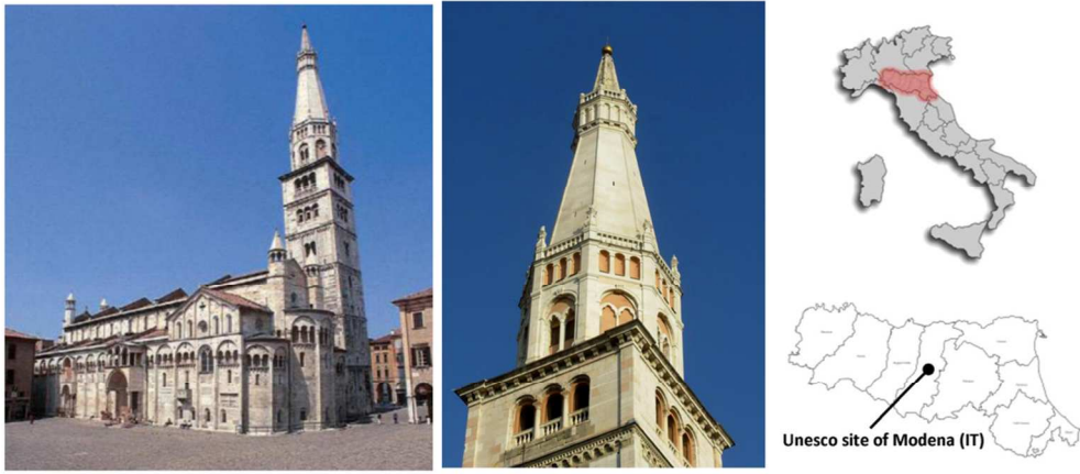
The Ghirlandina Tower and the nearby Cathedral, Modena (Italy), included within the UNESCO World Heritage List since 1997 (left); detail of the top of the Tower (middle); location map (right). 105x47mm (300 x 300 DPI)
